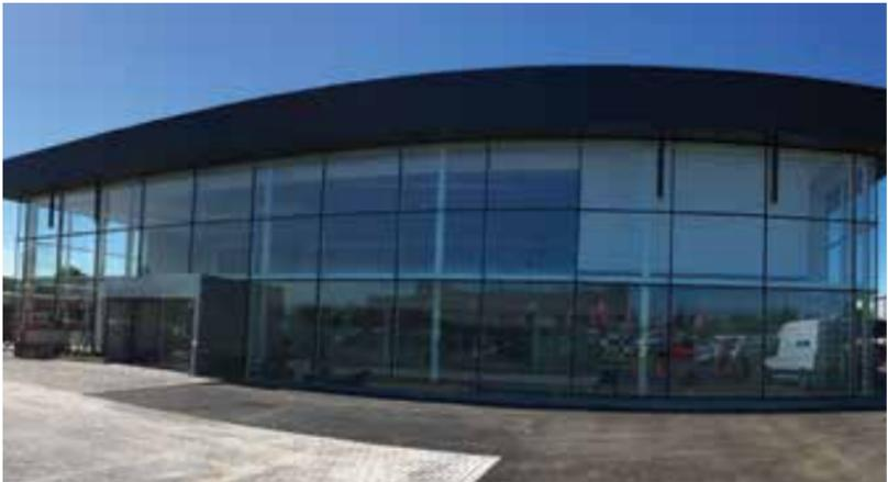
The steel frame building is clad to customer branding requirements with integral signage. A parapet encloses the roof, with an internal gutter, allowing for concealed rainwater pipes within the building. Both the main building and the valet bay building are supported on piled foundations.
